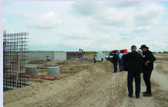
Touring the construction site for the new Sustainable Beef plant in North Platte, NE.
